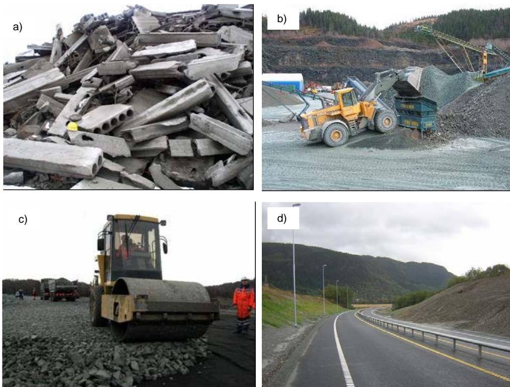
**Fig-3: a) Hollow core reinforced concrete waste was used to produce recycled aggregates b) Cushing and sieving to particle sizes of 0/100 mm and 20/100 mm c) Paving and compaction of sub-base material after sprinkling d) Finished test section of the highway E6 Melhus (Aurstad et al., 2005)**
