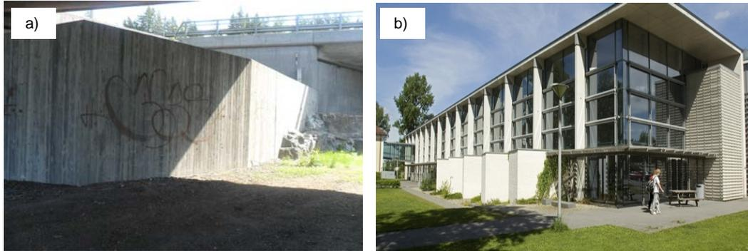
**Fig-2: a) Concrete retaining wall with recycled coarse aggregate content of 780 kg/m<sup>3</sup> (Highway E6, 20 km south of Oslo, Norway) b) Concrete foundations, columns and basement walls with recycled aggregate content of 269 kg/m<sup>3</sup> (Sorumsand High School, Norway)**
