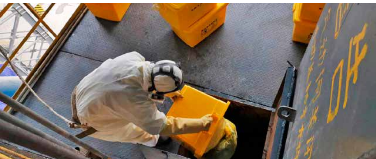
7 Covid-19 hospital and health care wastes emptied from the hard-plastic box directly into the kiln-inlet at 1 t/h
