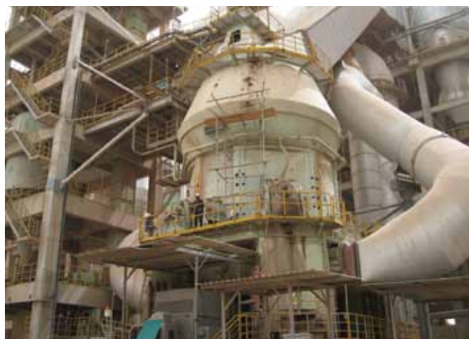
Figure XX.2: feeding of waste-derived mineral additions to the cement mill
