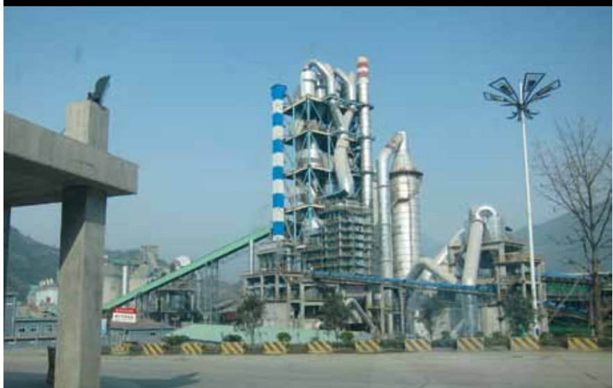
Cement plant by the Yangtze River in China
